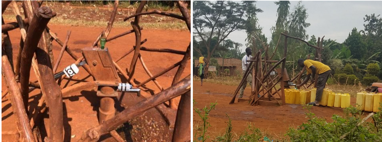
Figure A11.7. Borehole 1 near Jinja.
