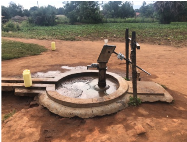
Figure A11.12. Borehole 3 in Gulu.
