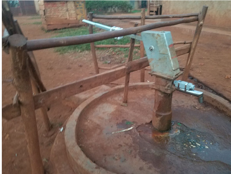
Figure A11.11. Borehole 2 near Jinja.
